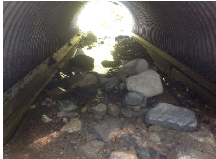
looking through culvert from inlet
